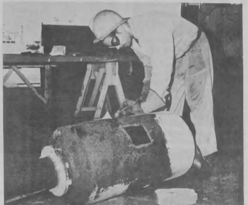
WHEN USING cutting torches, special goggles protecting against rays and chips are used. ORA TA usa torch di corta, bril special pa proteha contra rayo y chip di heru ta usa.
